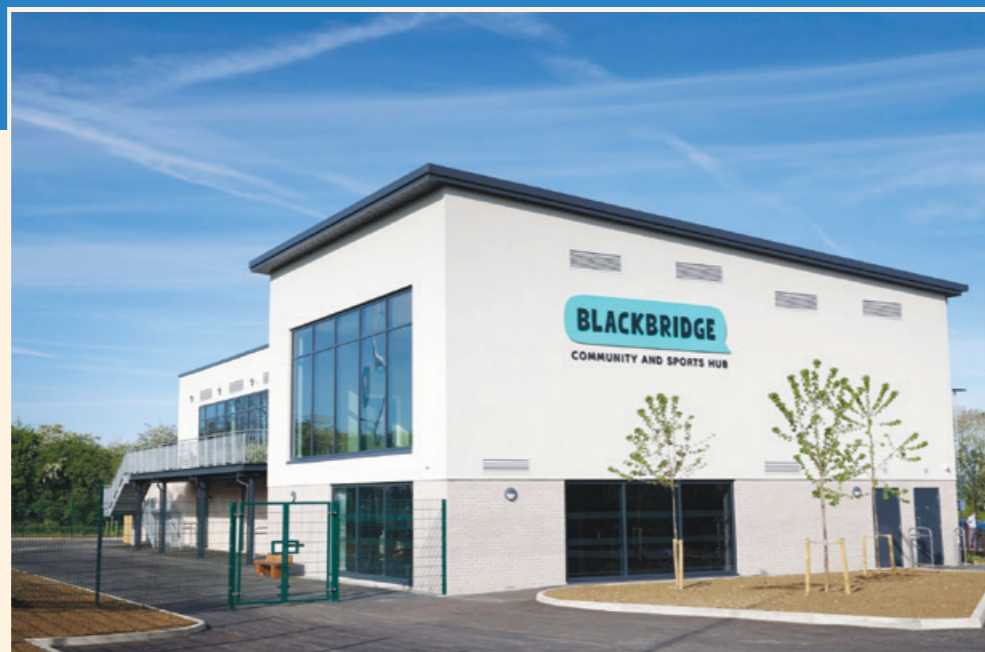
Open for business: The new Blackbridge Community and Sports Hub
